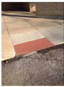
Grade B – Minor Deficiency: The curb ramp shown on the left lacks required turning space.
