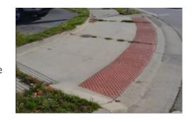
Grade D – Multiple Major Deficiencies: The curb ramp shown on the left does not have a detectable warning, does not have the required running slope and turning space, and is overgrown.
