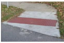
Grade C – Major Deficiency: The curb ramp on the right does not have the required running slope, is overgrown, and the detectable warning is worn out. Curb ramps with no detectable warning automatically receive a grade of C.
