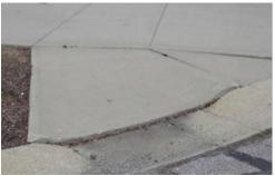
Grade F – The ramp on the right does not have a curb ramp. The ramp on the left is broken and impassible.
