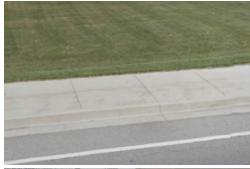
Grade B – Minor Deficiency: The sidewalk shown on the left has a bad cross slope and is slightly overgrown.
