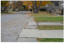
Grade D – Multiple Major Deficiencies: The sidewalk shown on the left is too overgrown, narrow, contains lots of level changes, and has a bad cross slope.
