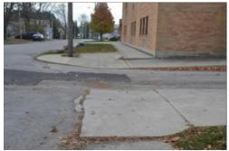
Grade C – Major Deficiency: The sidewalk shown on the left has a bad cross slope, is very overgrown, and has abrupt level changes making it difficult to navigate by wheelchair, but still passable for someone walking.
